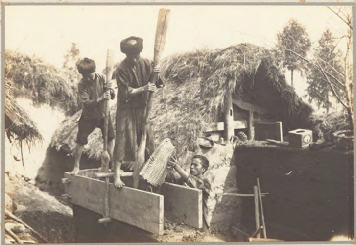
Building mud walls— when kept well covered with grass or straw or tiles, they stand for many tens of years.
