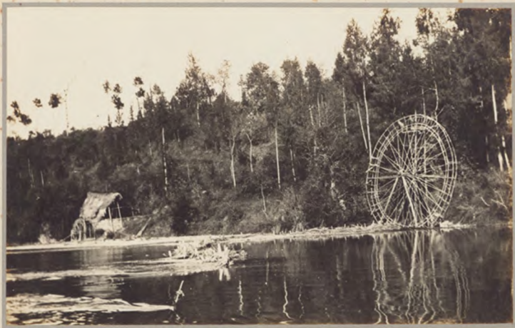
A 'Bamboo' irrigation water wheel—conveys water some tens of feet high up, to supply water for the rice paddy fields. It is driven by the running river water.
